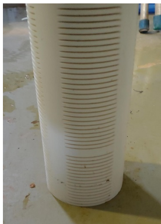
Image 5-11. Hatchery ER Floor Drain Covers (1.0 mm)
