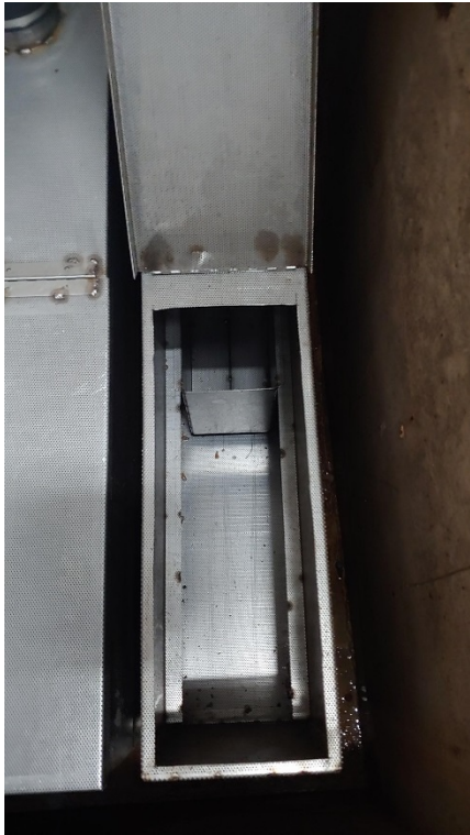
Image 5-25. 1.5 mm Stainless Steel Containment Baskets Located in the Hatchery Main Containment Sump
