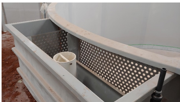
Image 5-28. Water exiting the AR tank side boxes flows through a second 25 mm screen on the way to the RAS drum filter.
