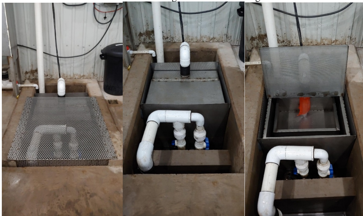
Image 5-17. Hatchery ER Containment Sump and Stainless Steel Containment Baskets
