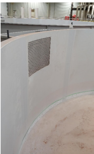
Image 5-27. 25 mm screen installed in AR tank walls over the side box opening.
