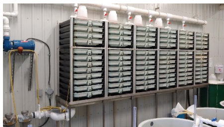
Image 5-1. Heath Stacks used to incubate eyed-eggs in the Hatchery and Grow Out Units.
